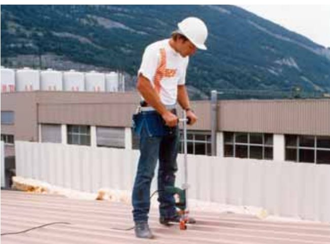
Assembly of trapezoidal sheet metal using self-tapping screws
