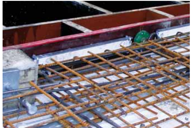
Installing HALFEN HTU Cast-in channels in the front-face of a slab
