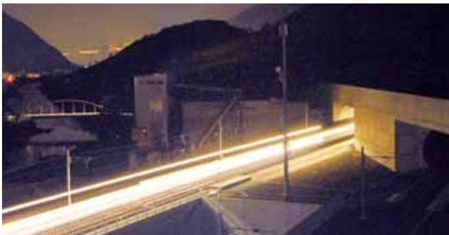
Lötschberg-Base tunnel, Switzerland
