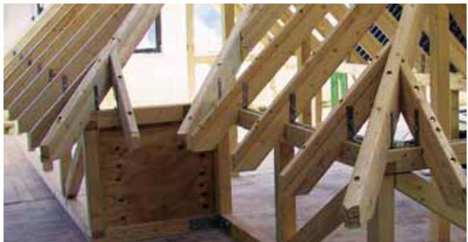
Timber pitched roof construction
