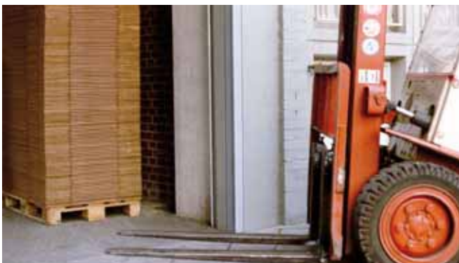
Corner guards in an industrial environment
