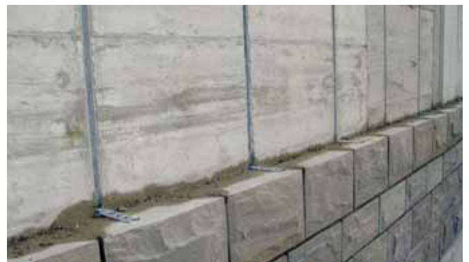
HALFEN ML Brick-ties anchor system
