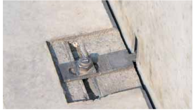
HALFEN HKZ Restraint tie with serrated washer
