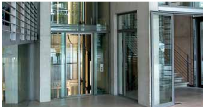
Lift fixings, guide rails
