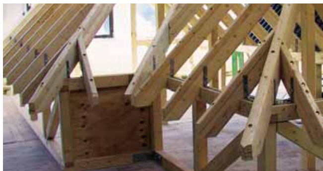
Timber pitched roof construction
