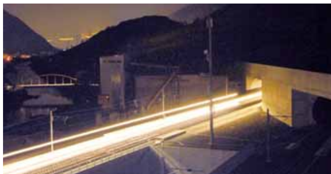
Lötschberg-Base tunnel, Switzerland
