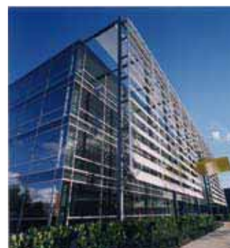
Peoplebuilding Hemel, UK
