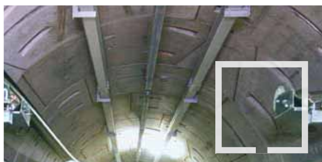
Sine HALFEN in elemente Tübbing
